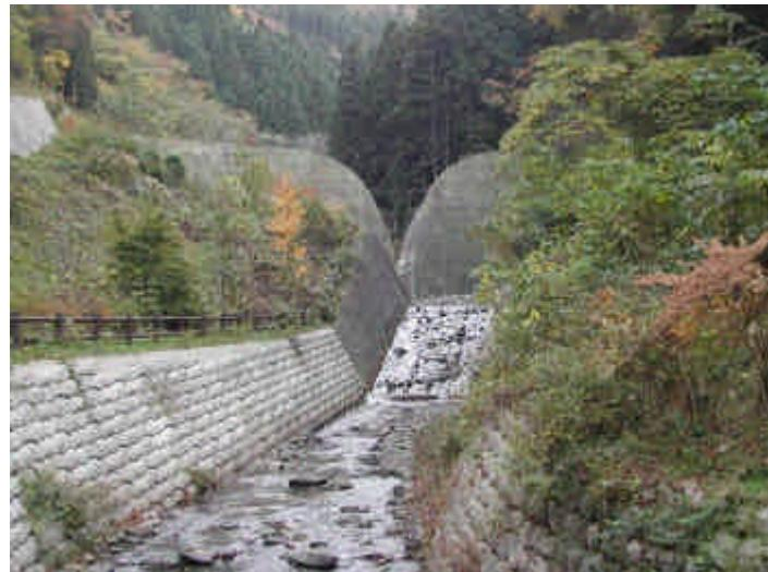
The slit sabo dam and protection wall
