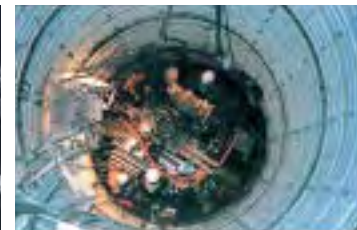
集水井工 Drainage well works
