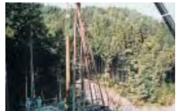
杭工 Piling works
