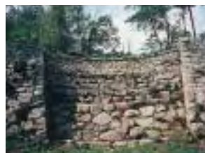
圭峰砂留 Keiho sunadome (the sabo dam at Keiho)
