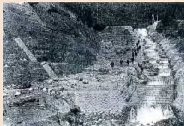
▲施工直後（1920年代） Immediately after works (1920's)
