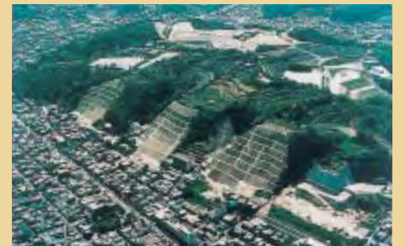
対策工施工直後 Immediately after the completion of the works
