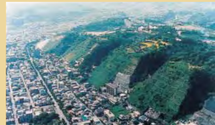
施行後数年経過 Several years after the completion of the works
