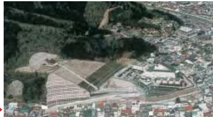
施工後 (After the completion prevention works)
