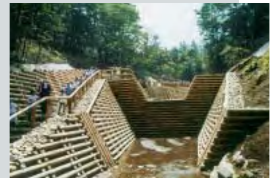
Ground sill works (Mt. Hachimantai)
