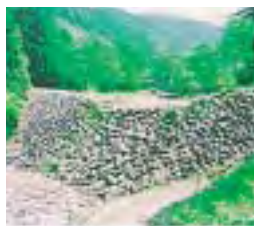
岐阜県南濃町「般若谷」の巨石えん堤 A dam built with big stones at "Hannyadani," Nanno Town, Gifu Prefecture
