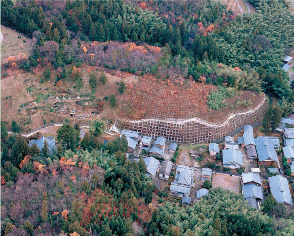
Igake area (Niigata City) Construction: 1998 - 2005
