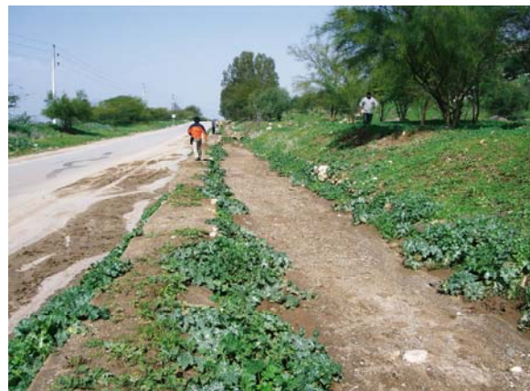
Photo-1 Damage of road north of the Dead Sea
