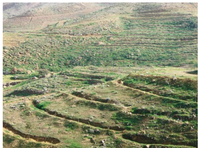
Photo-4 Contour terrace method on the slope of Jordan Valley
