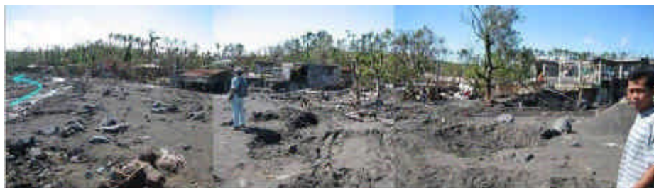
Photo.6 Damage at Daraga Town(1)
