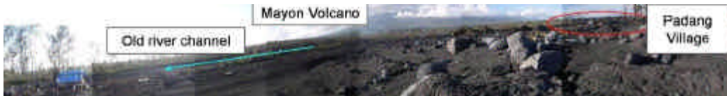
Photo.3 Damage at Padang Village(2)
