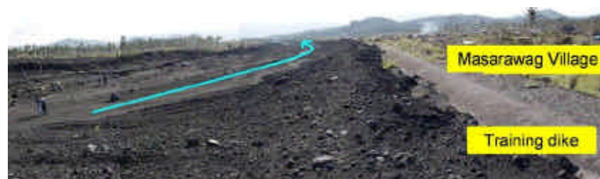
Photo.1 Damage was alleviated by training dike.
