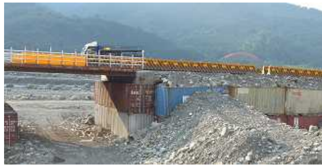
Photo-2: Temporary bridge abutments making use of container boxes
